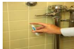
Wall area around toilet
